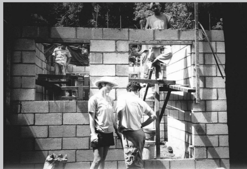
A Habitat for Humanity home under construction. When finished, the houses are about 130 feet in diameter. This three-room house is made of cinder block and will have a metal roof.
